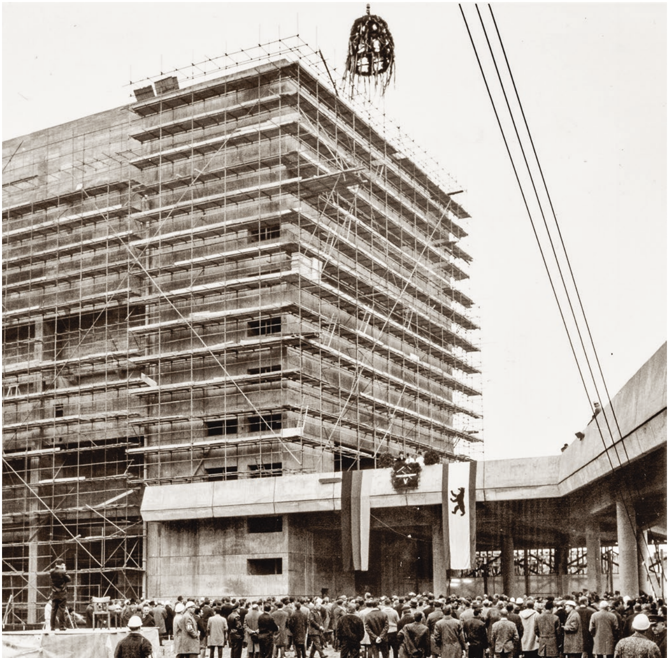
Roofing ceremony at the waste-to-energy plant
